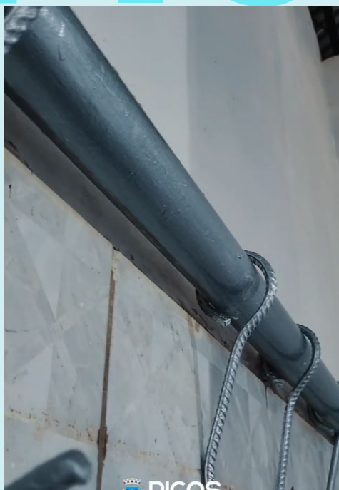
Reforma do Matadouro Municipal
